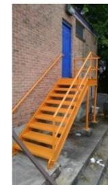
During the spring semester, our metal stairwell received new step plates, and a new surface plate. Another handrail was added. The stairwell also received a new paint job. The new plates should last another 30 years.
